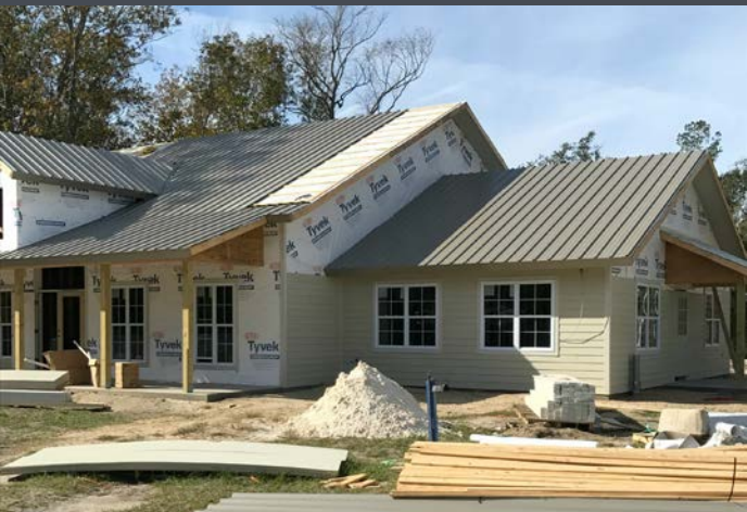
The new Counseling & Support Services Center at the Ranch.
